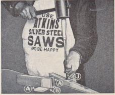
Fig. 25—Beating out mortise. Spalls A sawed from cheeks of tenon B, as shown in Fig. 14
