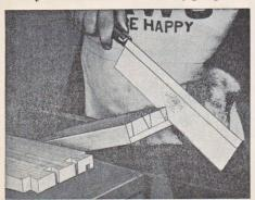
Fig. 29—Sawing half-blind dovetails with ATKINS Silver Steel Dovetail Saw
